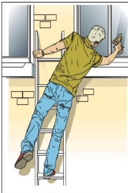
Overreaching – not maintaining 3 points of contact Do:
